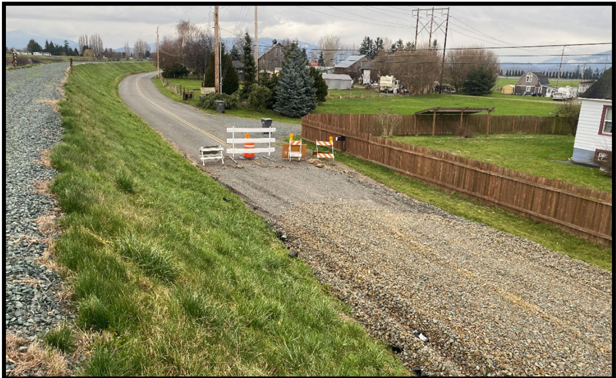
Photograph 2. View of the seepage berm placed at STA 121+00 on the landward side of the DD 17 levee during the November 2021 flood event.
