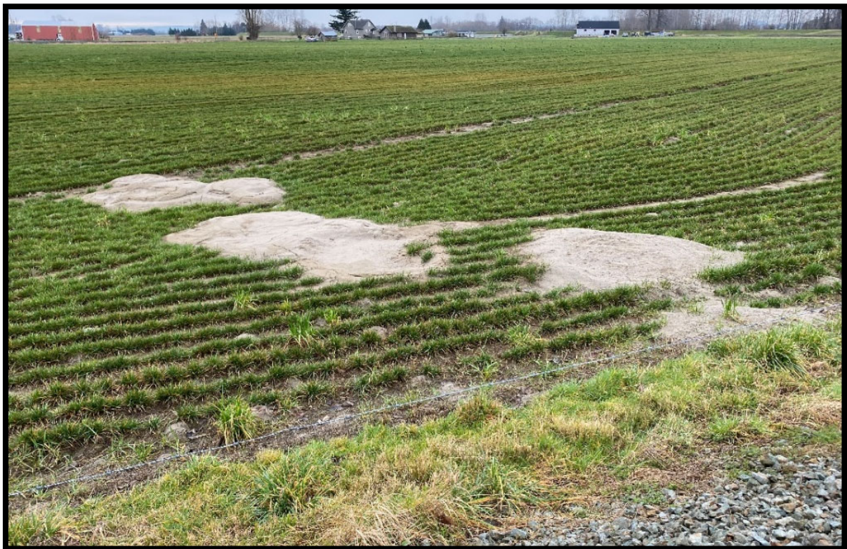
Photograph 4. View of Sand boils near the landward toe of the DD 22 levee at STA 357+00.
