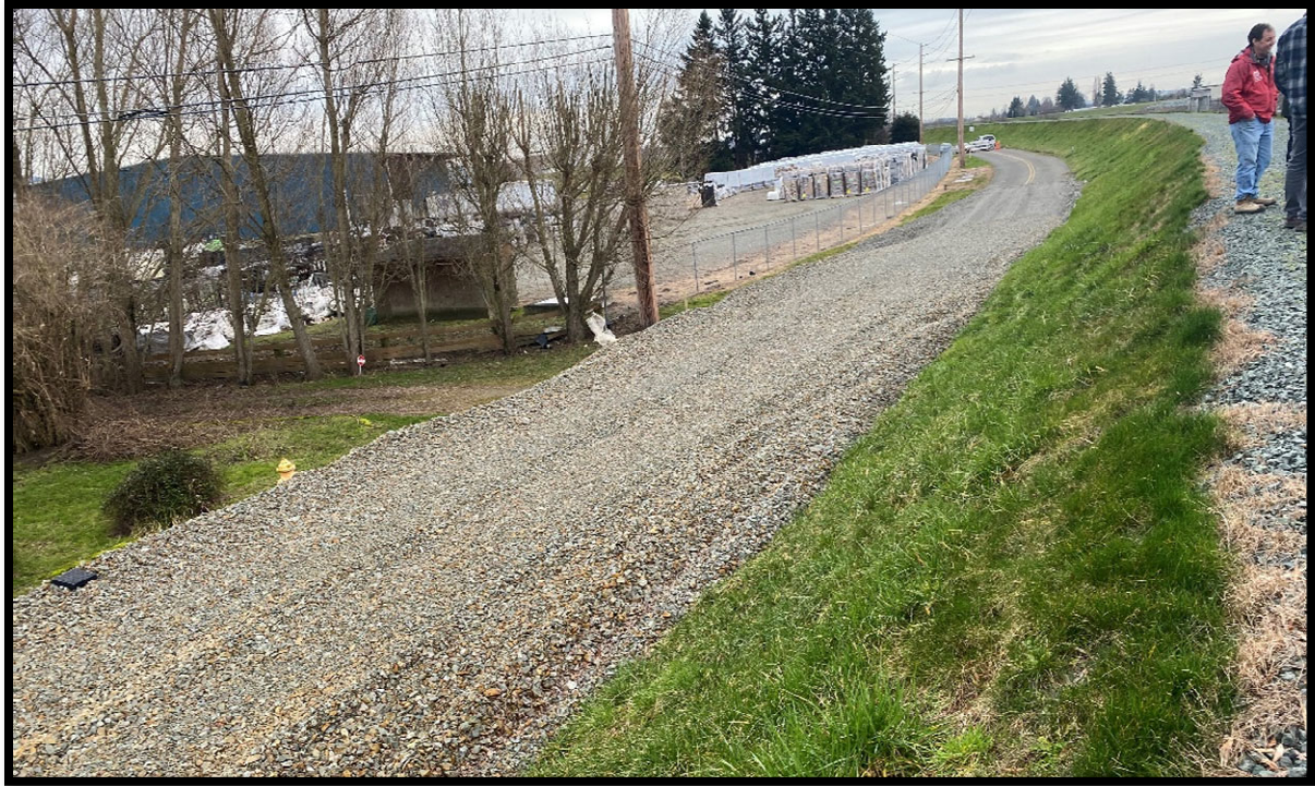
Photograph 3. Typical landward slope of the DD 17 levee, upstream oriented near STA 120+00. The seepage berm was placed on the landward side of the levee during the November 2021 flood event.
